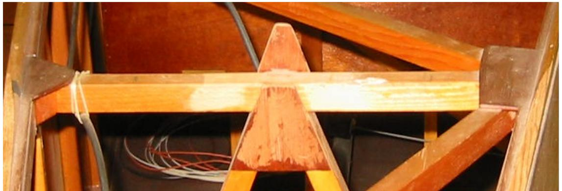
**Figure 3: Reinforced Truss Joints (Nordin, 2006)**
