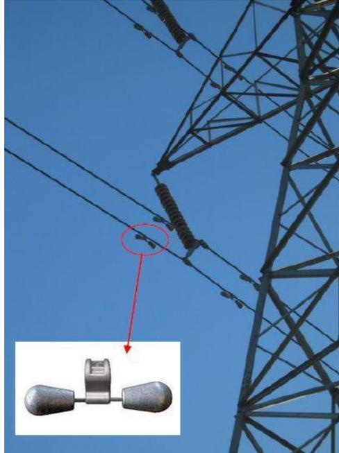
**Figure 5.3: Power line vibration absorber [49]**
