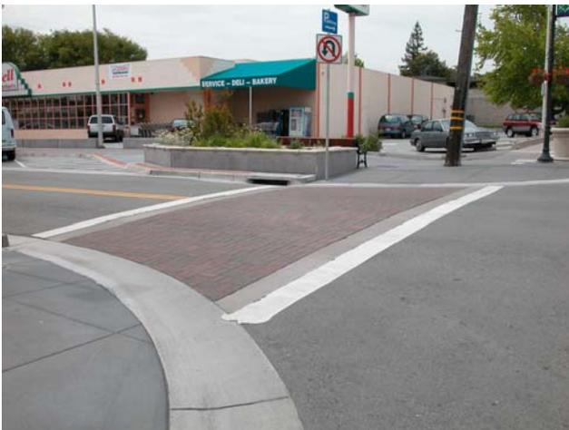
Figure 16. Example of raised sidewalk
