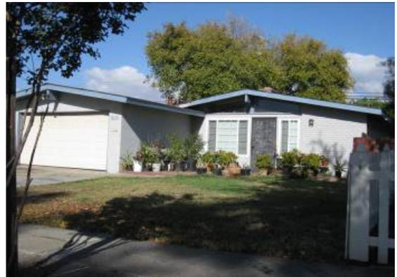
**Figure 25 Flat or Minimally-Sloped Roof**
