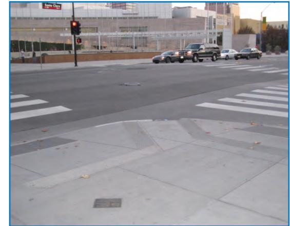
Figure 4.19 Example of a dual curb cut with detectable warning material
