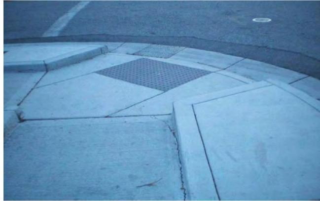
Figure 22 ADA Compliant Ramp
