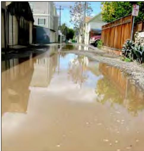
**Figure 3.3:** Alley with Poor Drainage.
