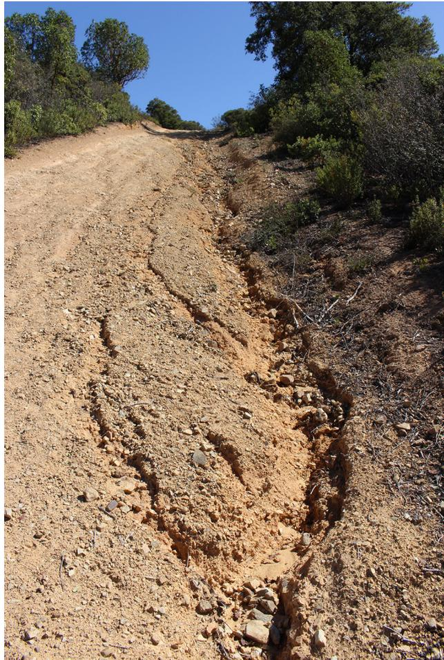
Figure 3.1. Erosion along the Priest Rock Trail in the Sierra Azul OSP.
