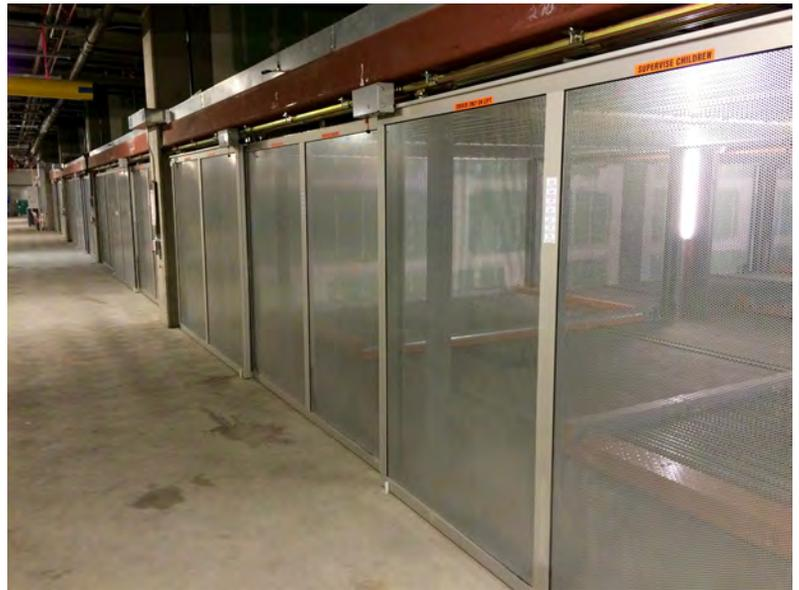
**Figure 5.1: Stalls with mechanical stackers.** Such parking arrangements are becoming a more common and accepted way to meet parking requirements without adding another complete underground level.
