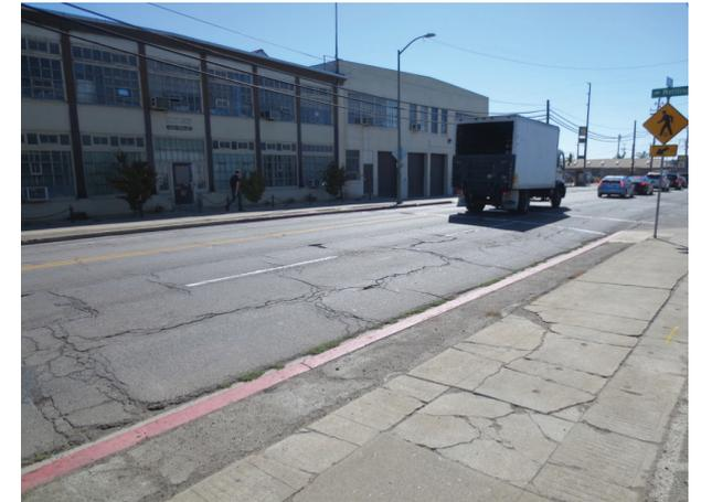
Figure 18 - Poor Pavement Conditions near Watling St.
