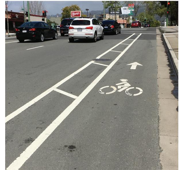
Figure 43 - Buffered Class II Bike Lane on Broadway - Oakland, CA.
