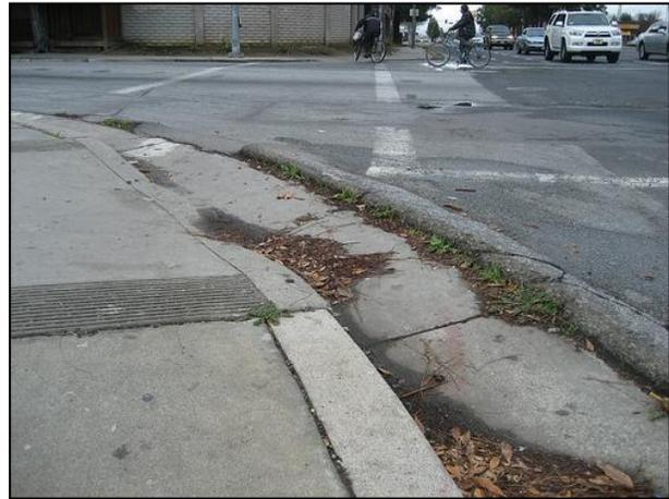
Figure 46. Buckled asphalt at curb ramp.
