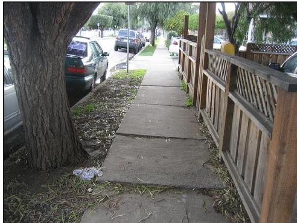
Figure 34. Sidewalk in poor condition.
