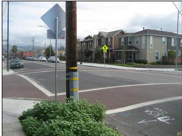
Figure 51. Colored crosswalk paving material.
