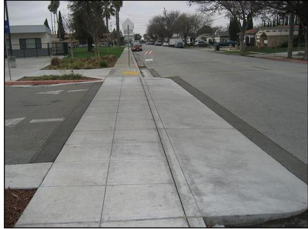
**Figure 49. Driveway with sidewalk material extended over it.**
