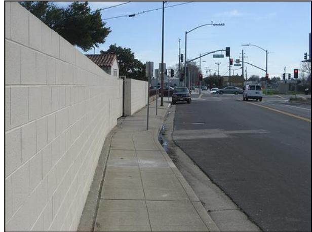
**Figure 39. Monolithic sidewalk.**
